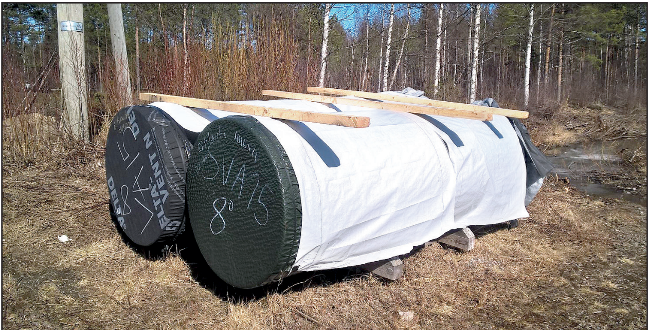
Figure 5. Pipe ends protected by plastic covers, black pipe fittings protected with white cover against sun heat in summer
